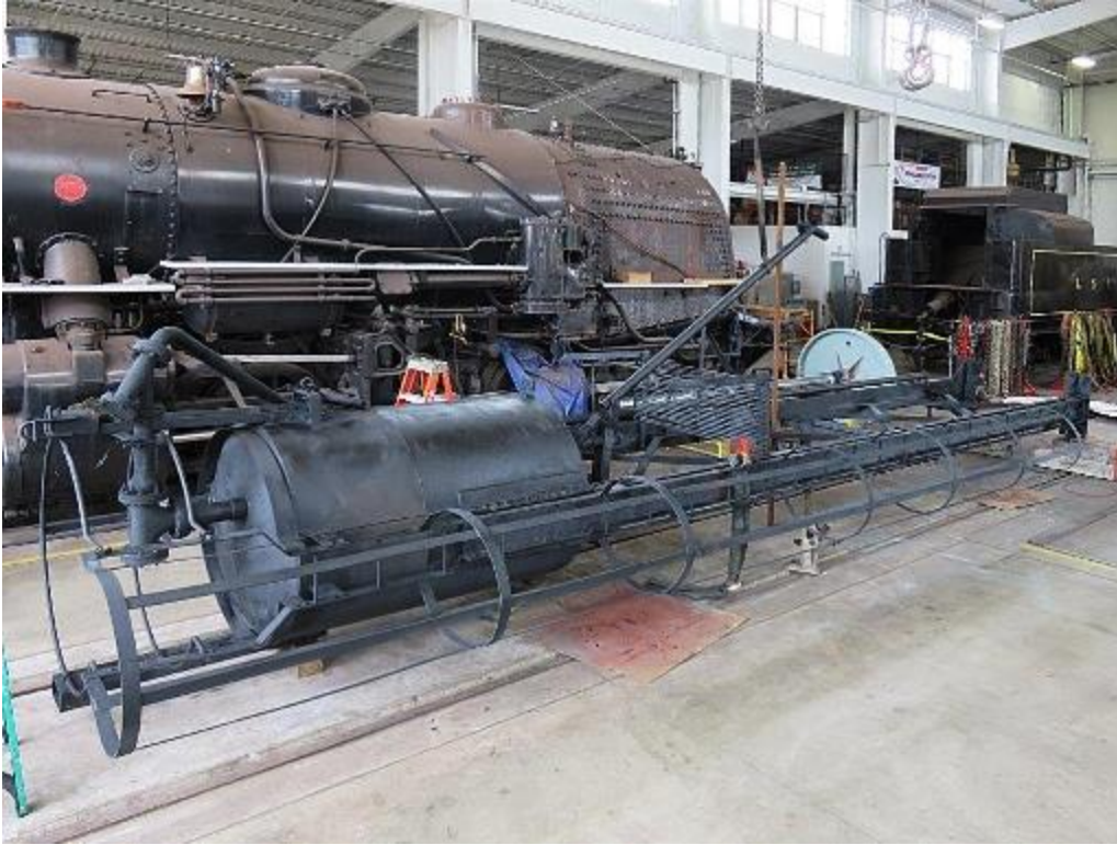
Former AC&Y sand tower being prepared for installation
