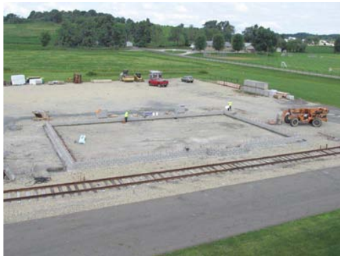
Admin/Office Building Foundation
